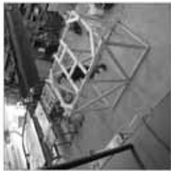
4. Frame assembled at the shop.
