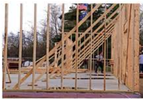
Softwood Lumber Bracing
