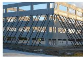
Tilt-Up Concrete Bracing
