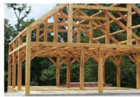
Heavy Timber Framing
